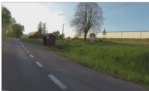
Fig. 13 Risky implementation of the bus stop in rural areas (on the left km 47-46) and missing pavement in urban areas (on the right km 52-53)
