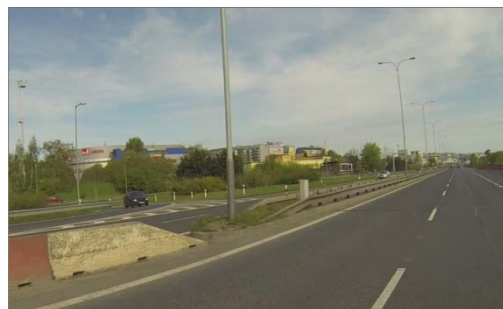
Fig. 8 Inadequate transition of road safety barrier in location no. 2, on the left km 17-18, on the right km 23-22
