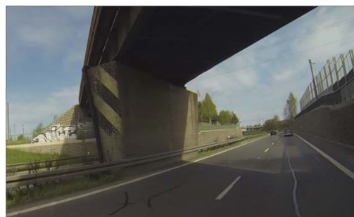
Fig. 11 Inadequate working width in location no. 3, on the left km 35-36, on the right km 31-30
