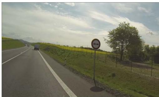
Fig. 7 Inadequate vertical and horizontal road signs prohibiting overtaking in location no. 1, on the left km 2-3, on the right km 7-6
