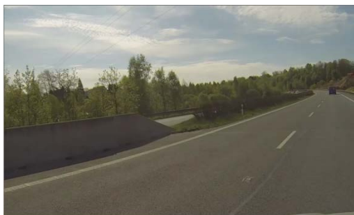
Fig. 8 Inadequate transition of road safety barrier in location no. 2, on the left km 17-18, on the right km 23-22
