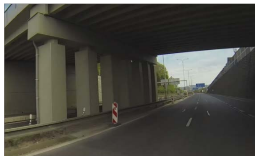
Fig. 9 Inadequate working width of road safety barrier - location no. 2, on the left km 18-17, on the right km 23-22
