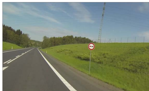
Fig. 7 Inadequate vertical and horizontal road signs prohibiting overtaking in location no. 1, on the left km 2-3, on the right km 7-6
