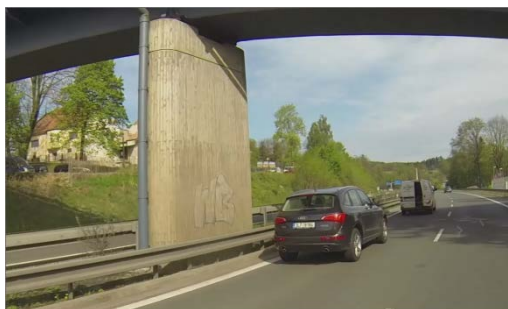
Fig. 9 Inadequate working width of road safety barrier - location no. 2, on the left km 18-17, on the right km 23-22
