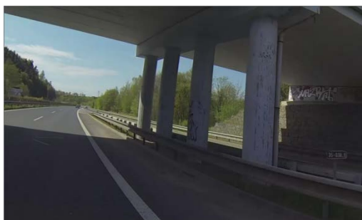
Fig. 11 Inadequate working width in location no. 3, on the left km 35-36, on the right km 31-30
