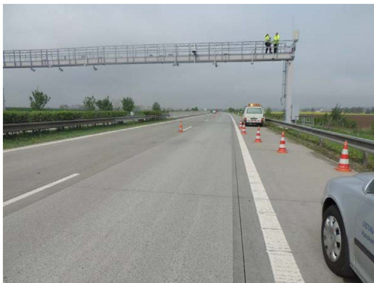
Fig. 9 Measured section of highway D1 [6]
